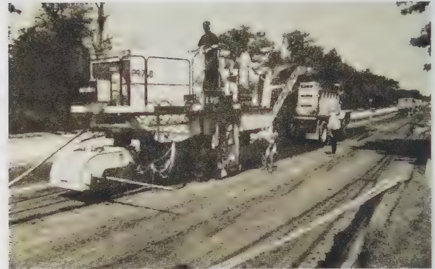
A pavement milling machine on Route 1. (1974)
